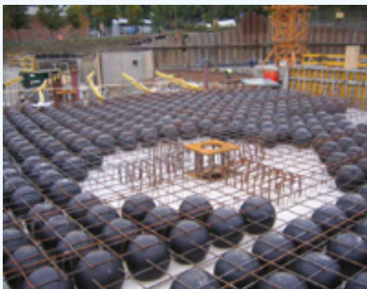
Figure 12: Use use of bubble-decks in building (Elkem)
